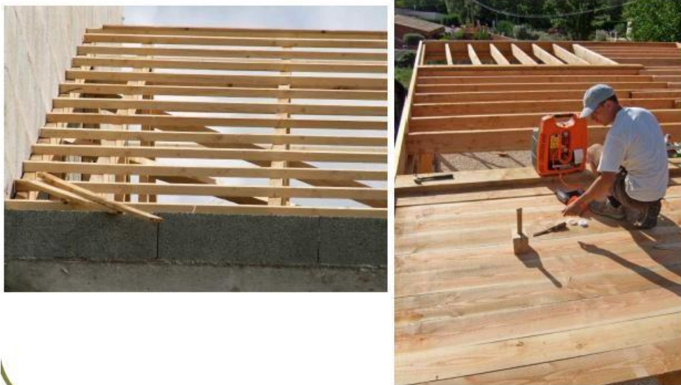
Figure II.21 Le support de couverture en bois [26].
